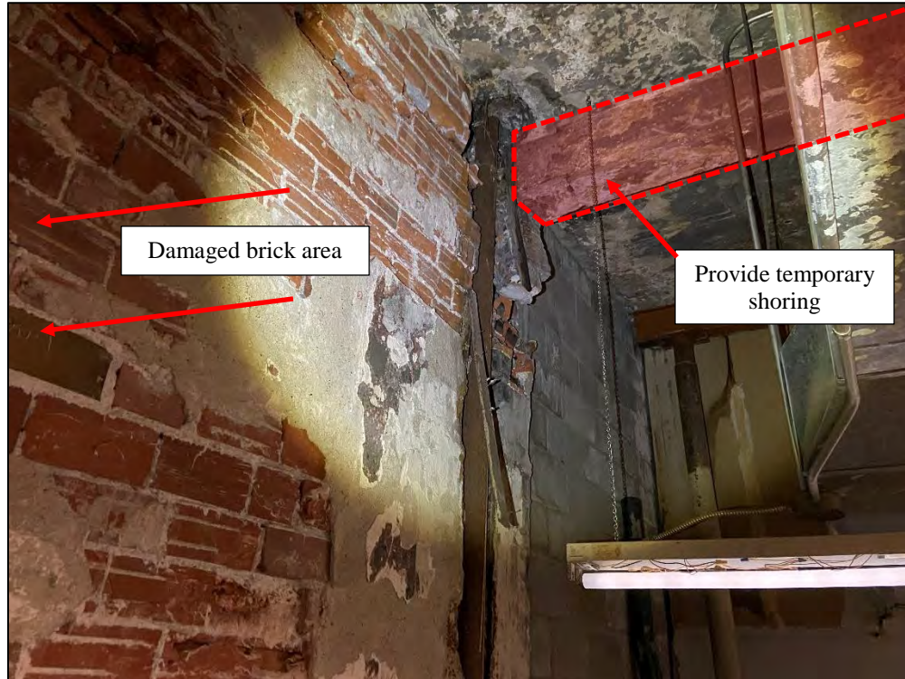
Photo 2 – Second Beam to Support
